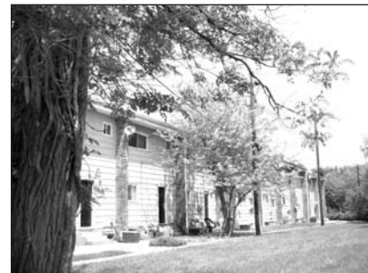
Catholic Charities' new family shelter is located in a residential area in Woodbridge, Virginia. Renovations of the building are scheduled for late summer and early fall. The front and back of the facility are shown above.
